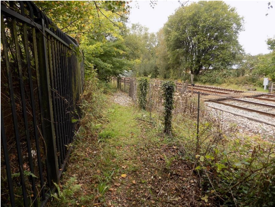
Figure 2-3.8: Up side approach to Wernddu Footpath Level Crossing
